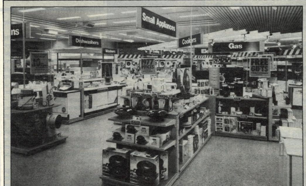
Currys' Stevenage superstore lit by low brightness fluorescent luminaires specially made for the project by Courtney Pope Lighting. The fully recessed fittings, each with two White 58W lamps, have louvres that give a wide light distribution. Average illuminance is 900 lux. The lighting creates a bright, airy atmosphere for the display of electrical goods while keeping energy costs to a minimum.
