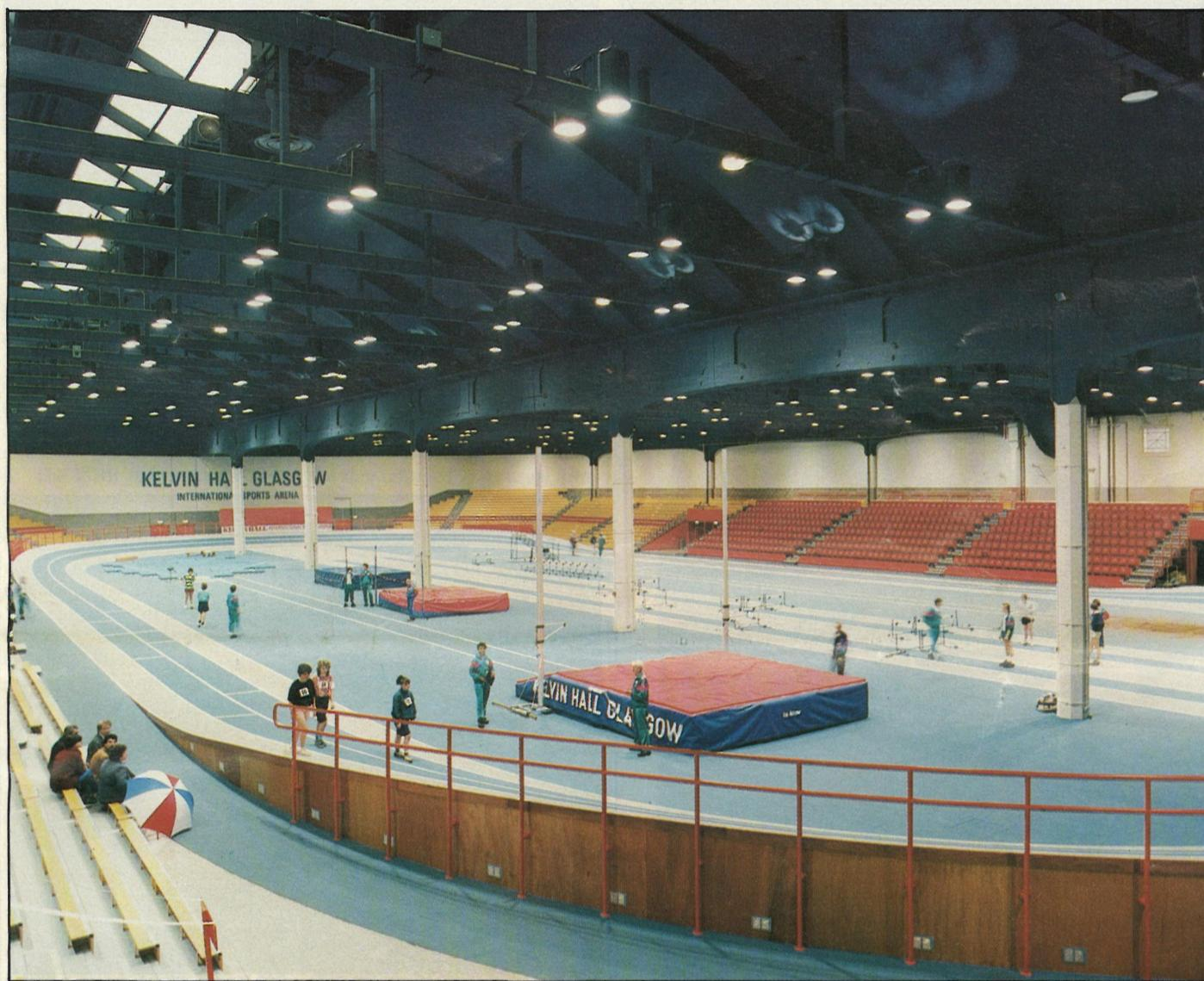
Metalarc was used in the Kelvin Hall indoor sports arena in Glasgow to provide the high levels of lighting — in excess of 750 lux — required for the televising of major events.
